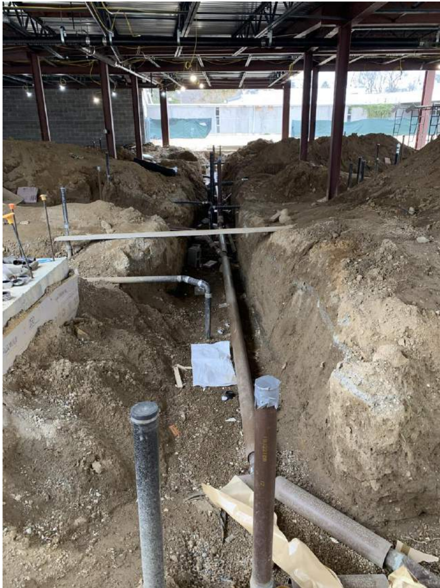
Jr/Sr HS New Addition Acid Waste Piping
